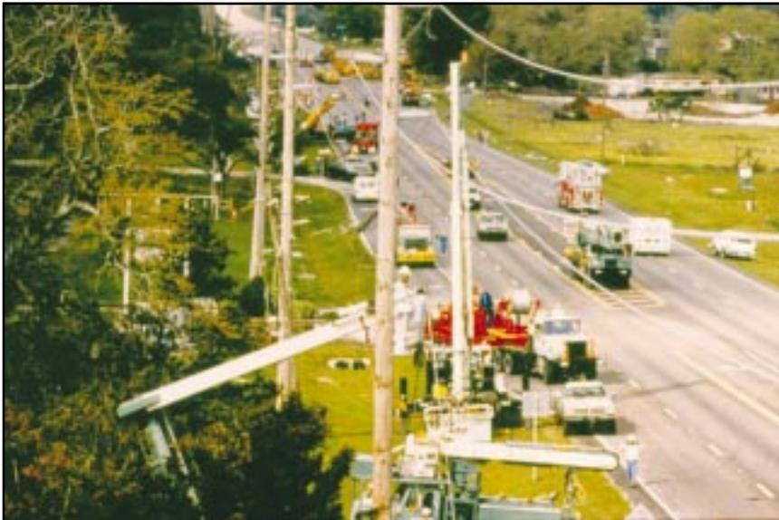
Replacing damaged poles and conductor along a busy right of way.
