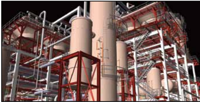
Figure 1: PDS is production-proven on small- and large-scale projects.
