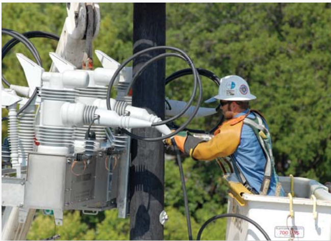
On the left, Oncor lineman Tim Lewis installs the IntelliRupter switch in the Dallas-Fort Worth area. On the right, the IntelliRupter PulseCloser switch is more groundbreaking technology that Oncor has installed in the development of its Smart Grid.
