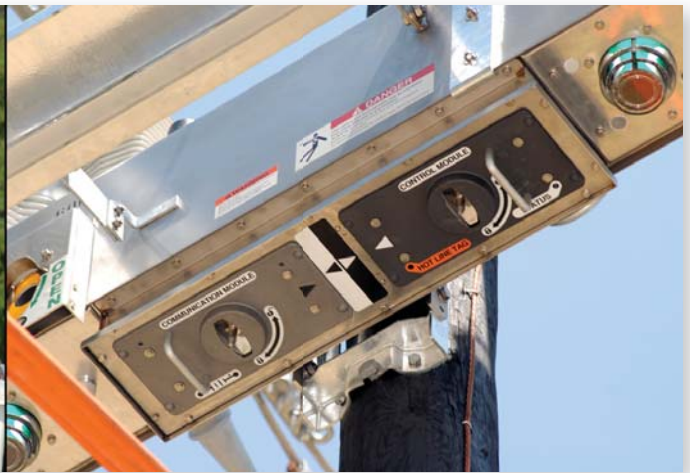
On the left, Oncor lineman Tim Lewis installs the IntelliRupter switch in the Dallas-Fort Worth area. On the right, the IntelliRupter PulseCloser switch is more groundbreaking technology that Oncor has installed in the development of its Smart Grid.
