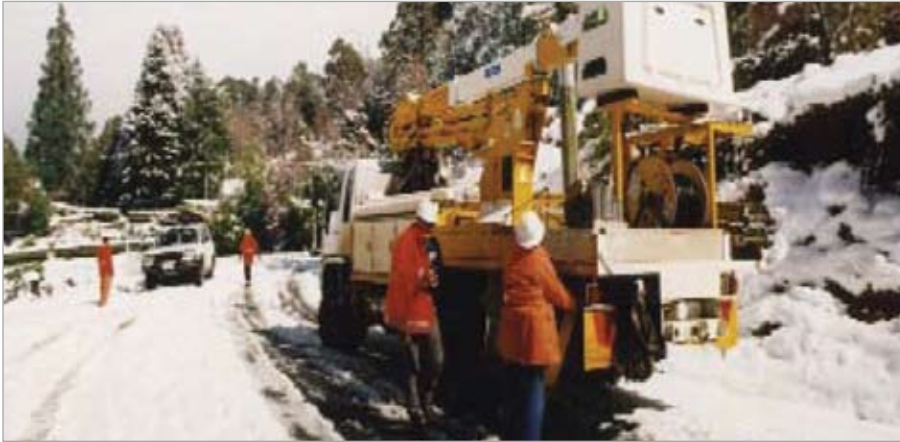
Aurora crews face the highs and lows of Tasmanian weather conditions.
